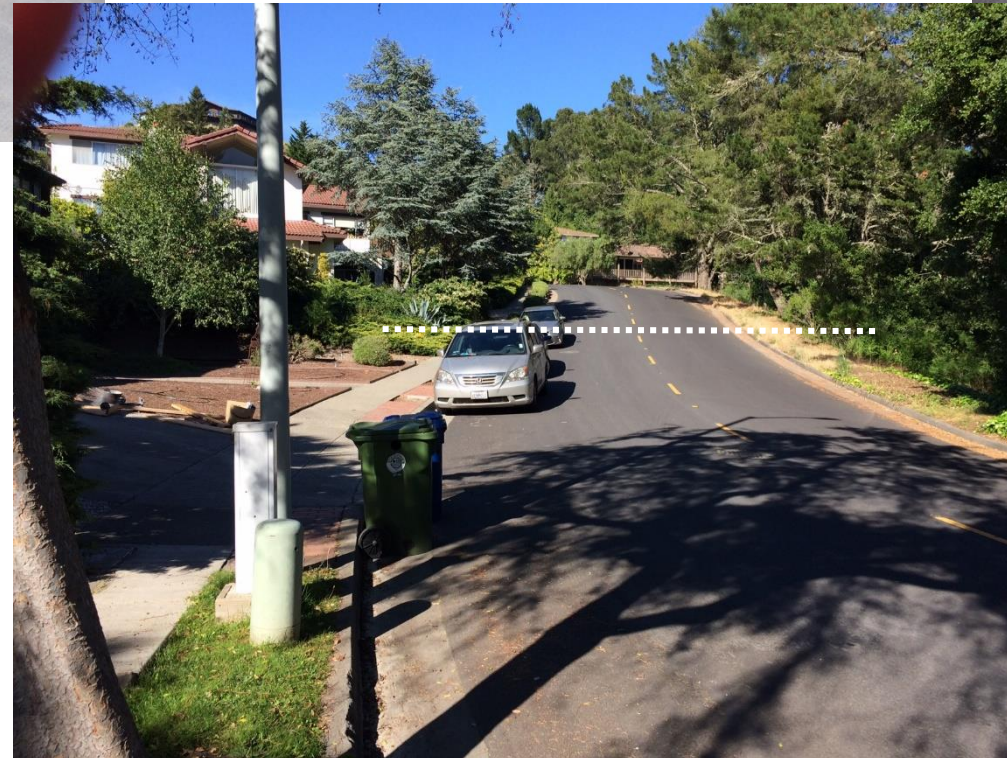
Hayward Fault scarp on Thors Bay Drive
